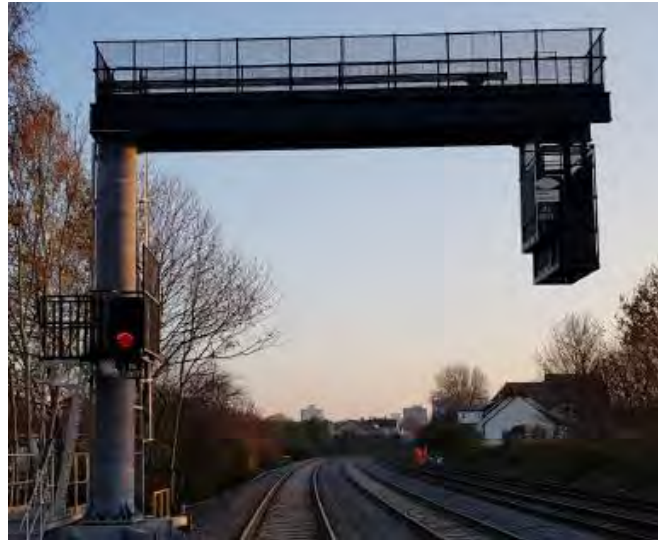
Figure 4-12 Sample cantilever signal gantry
