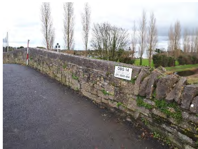
Figure 4-197 Existing parapet at OBG14
