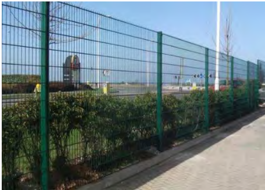
Figure 4-28 General purpose fence example
