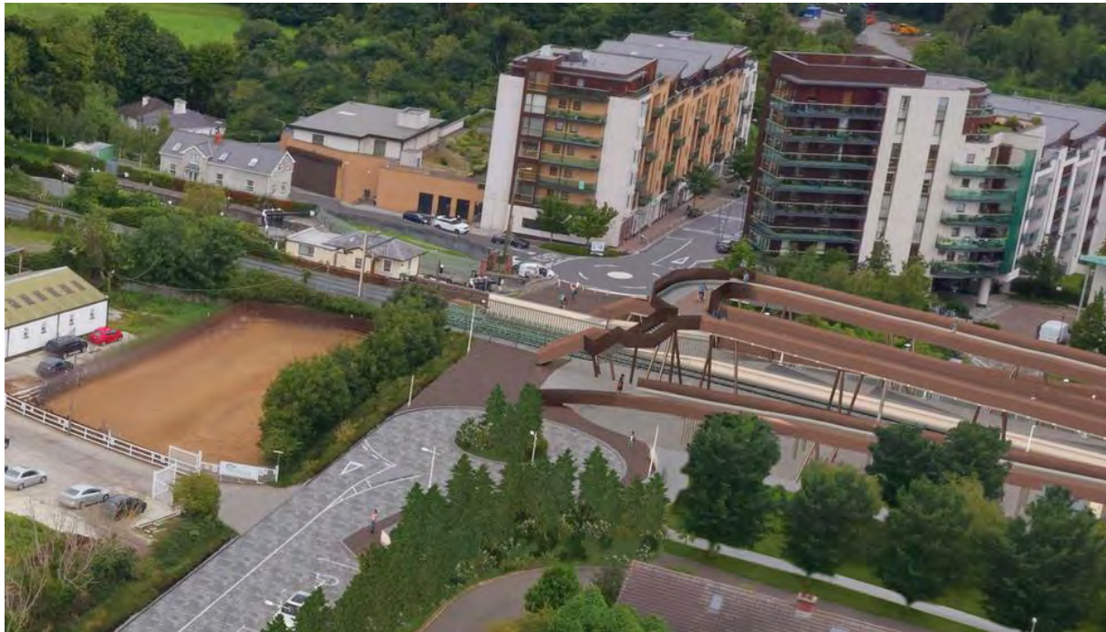
Figure 4-141 Ashtown Station after removal of level crossing
