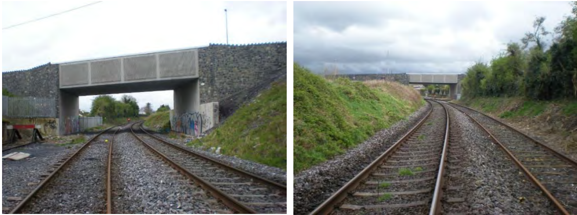
Figure 4-215 Left: siding to be converted into a running line. Right: siding with wood sleeper and without cant
