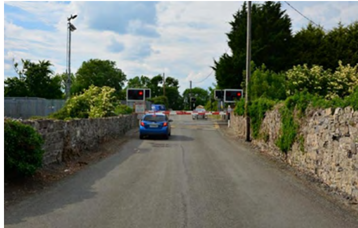
Figure 4-190 Barberstown level crossing
