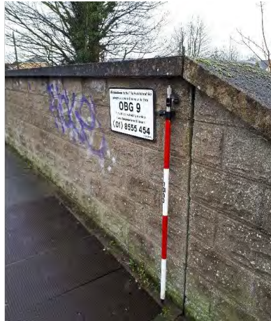
Figure 4-155 Existing parapet at OBG9
