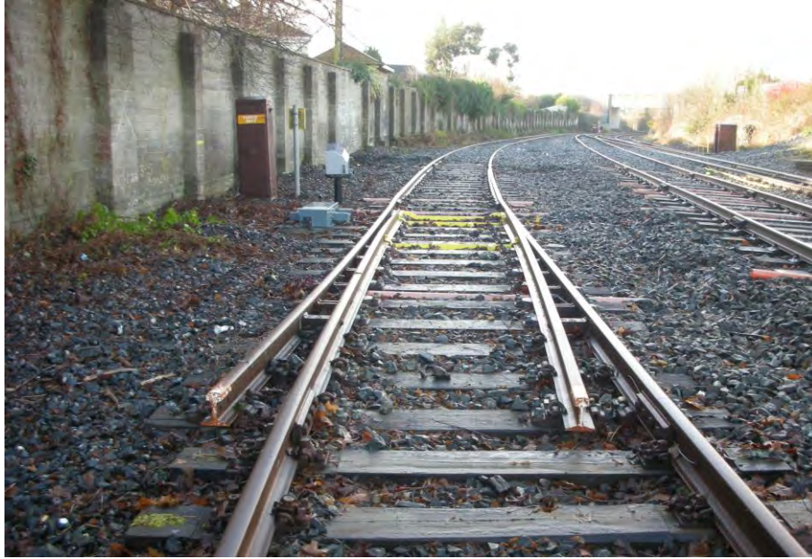
Figure 4-211 Current siding trap point. Source IAMS
