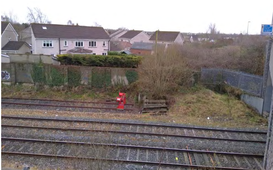
Figure 4-212 Current siding buffer stop. Source IDOM
