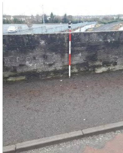
Figure 4-205 Existing parapet at OBG16
