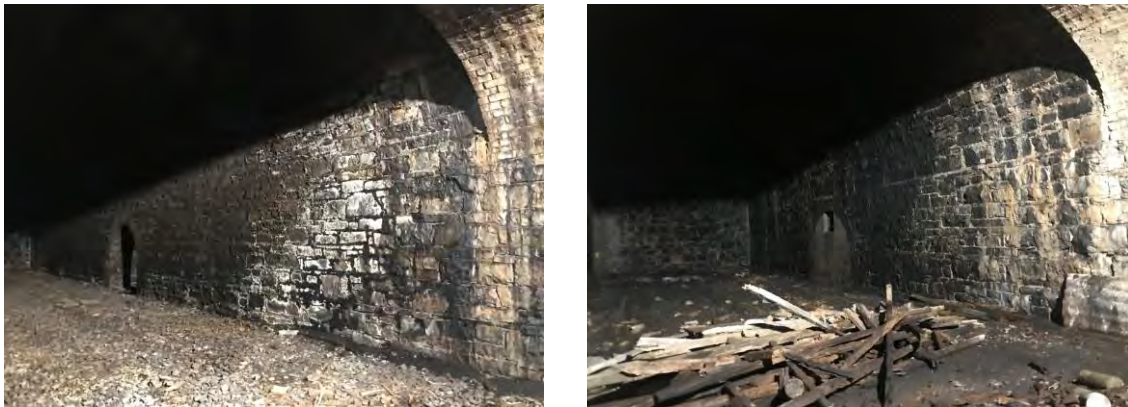
Figure 4-64 Current condition of the vaults
