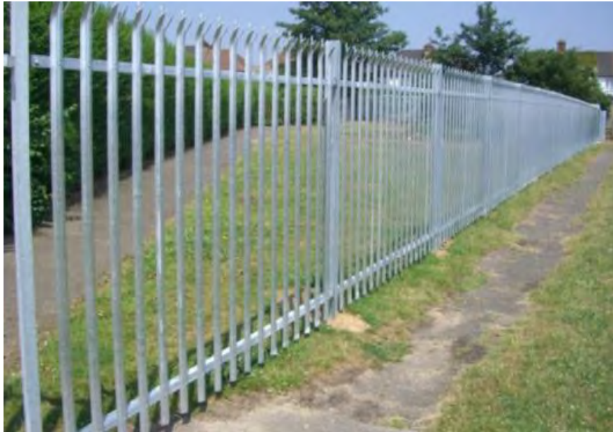
Figure 4-27 Palisade fence example
