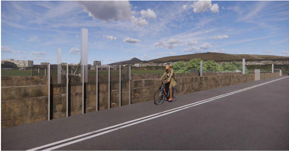
Figure 4-54 Wall heightening adjacent to catenary posts
